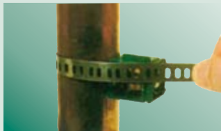
Cut mounting strip to length
