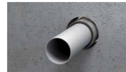
1. Slide the sleeve into the aperture and centre it
