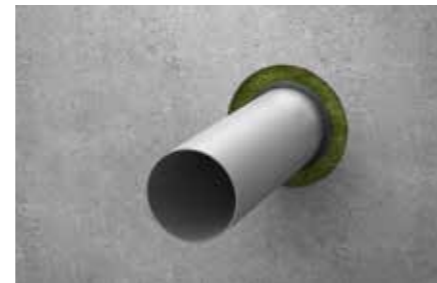
3. Close the gap between the wrap and the wall / floor with loose mineral wool.
