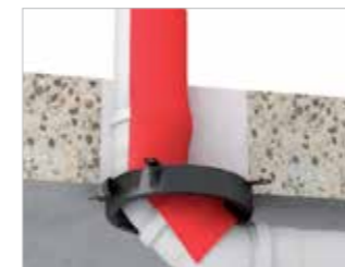
■ Bends directly under the ceiling
