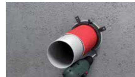
4. Drill (bending and sliding of fixing tabs is permitted)
