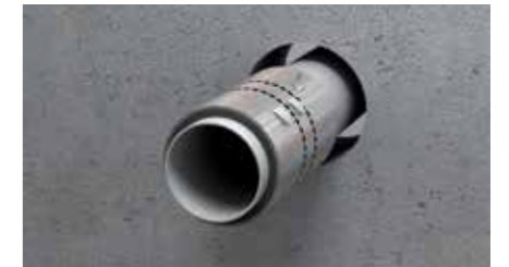
3. Bend and lock the tabs
