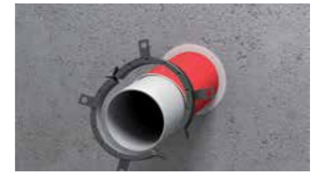
3. Select the correct collar size (in problematic built-in situations the use of an oversized collar is permitted up to max. 3 sizes bigger)
