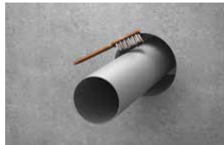
1. Clean the pipe and check the dimensions.
