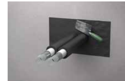
5. Flatten the Pacifyre® G with a jointing knife or trowel.
