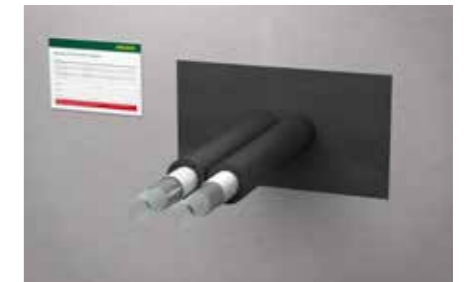
6. Place the filled out Pacifyre® ID-Card next to the penetration.
