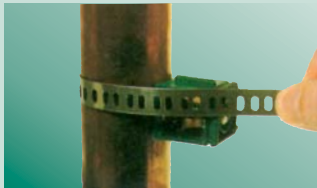
Cut mounting strip to length
