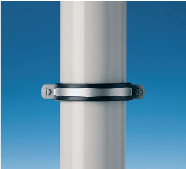
Figure 16: Pipe collar with rubber insert.
